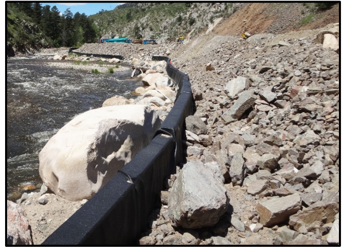
Concrete Barrier along Creek
