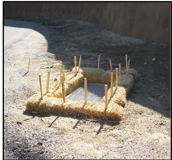
Erosion Bales installation around area inlets
