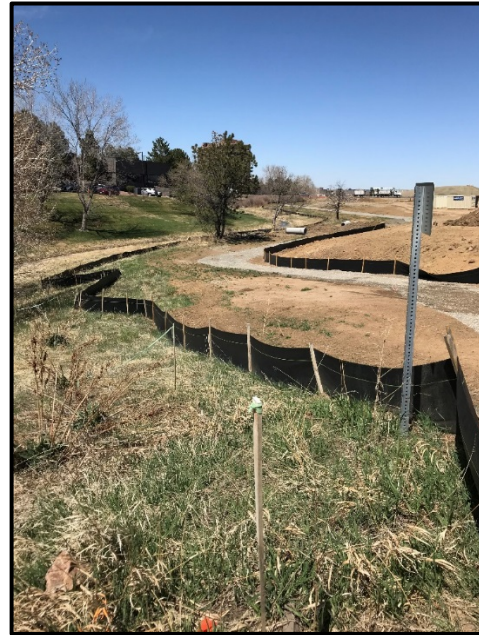
Stabilized Construction access road with secondary control measures
