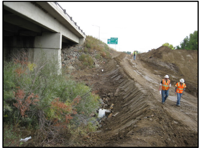
Temporary Berm along access road
