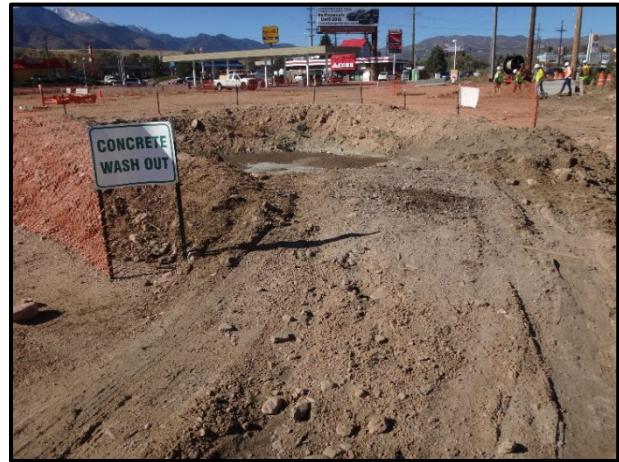
Concrete washout structure
