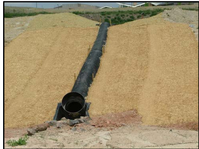
Temporary Slope Drain on stabilized slope
