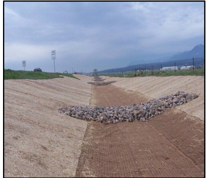
Rock check dam along lined drainage ditch
