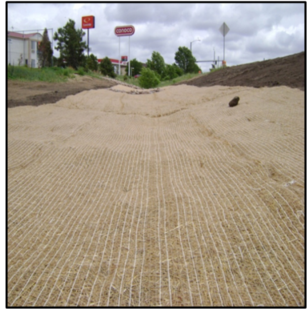
Soil loaded Turf Reinforcement Mat along drainage ditch
