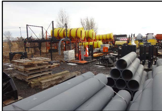
Site Waste and Materials Management
