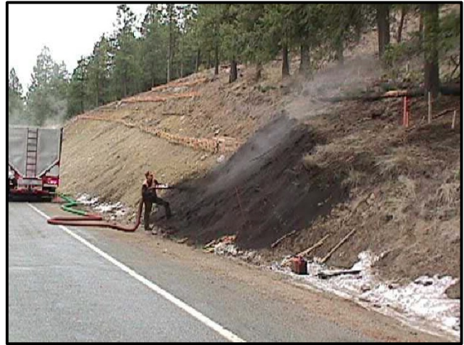
Compost Blanket Applications on Slope
