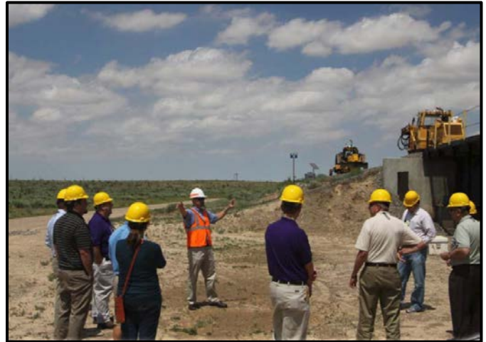
On site work coordination
