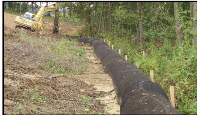
Brush Fabric Barrier - Credit West Virginia Department of Environmental Protection
